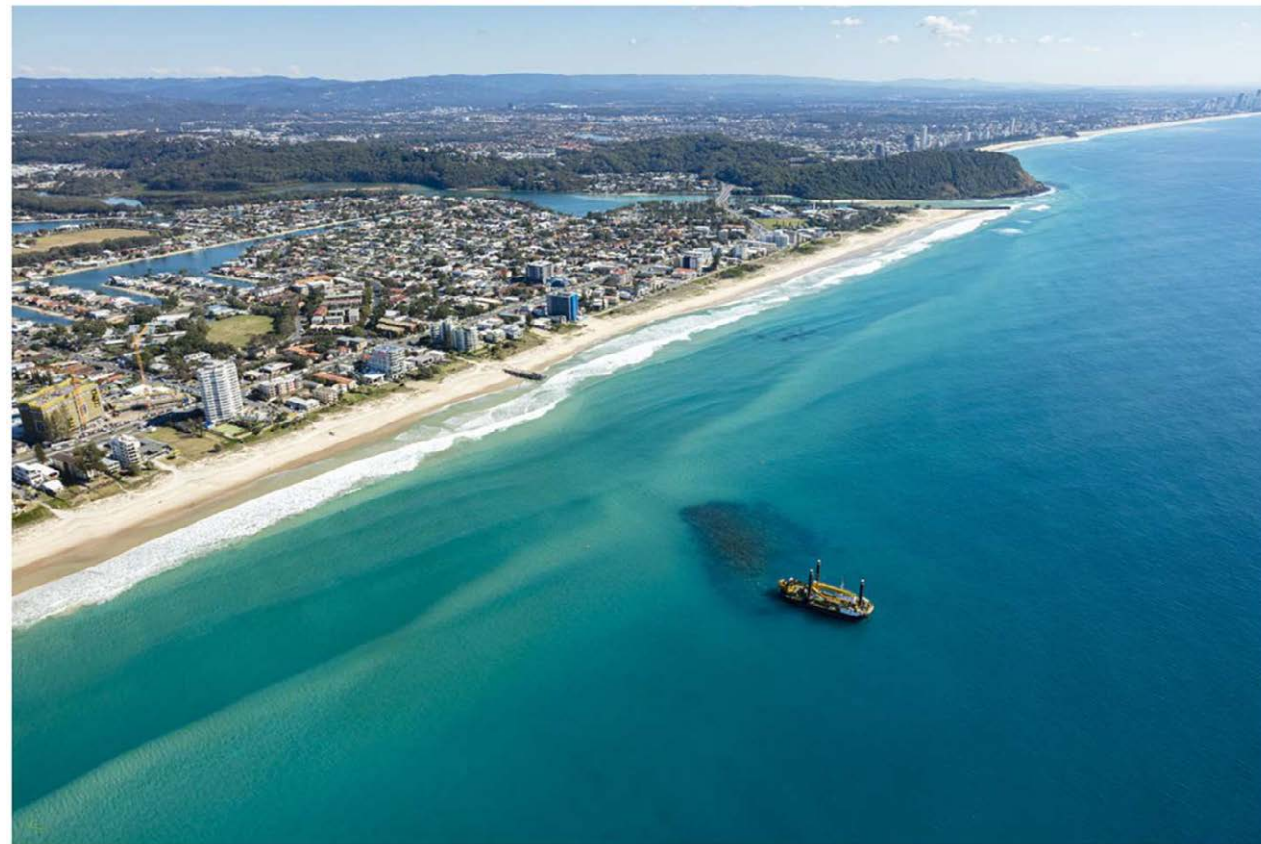
Aerial photo of the artificial reef construction
